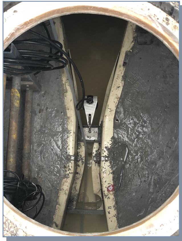
The picture above shows a Parshall flume with an ultrasonic sensor. The concrete is used for ballast weight, and to prevent stagnant water from developing in the sides of the flume. The flow meter automatically converts the level to a flow rate.
