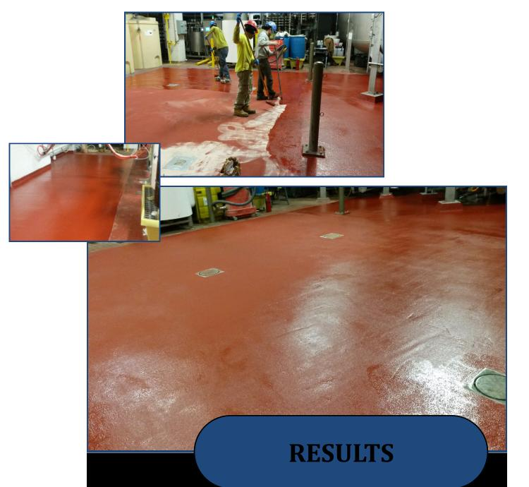
The finished floor provides greater structural support to withstand fork-truck traffic, is protected from chemical attacks, and offers improved slip resistance.
